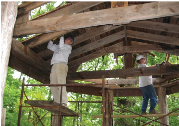
Steve Painter and Bill Daniel carefully remove rafters from the old roof.
